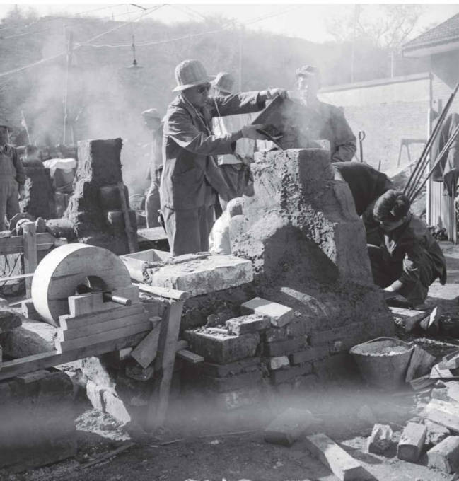
▲ Constructing a rudimentary smelting steel furnace, 1958
